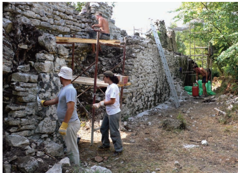
Conservation team consolidating the interior face of the Water Gate.
