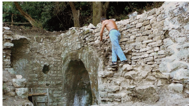
Building a dry stone wall to replace collapsed ancient walls.
