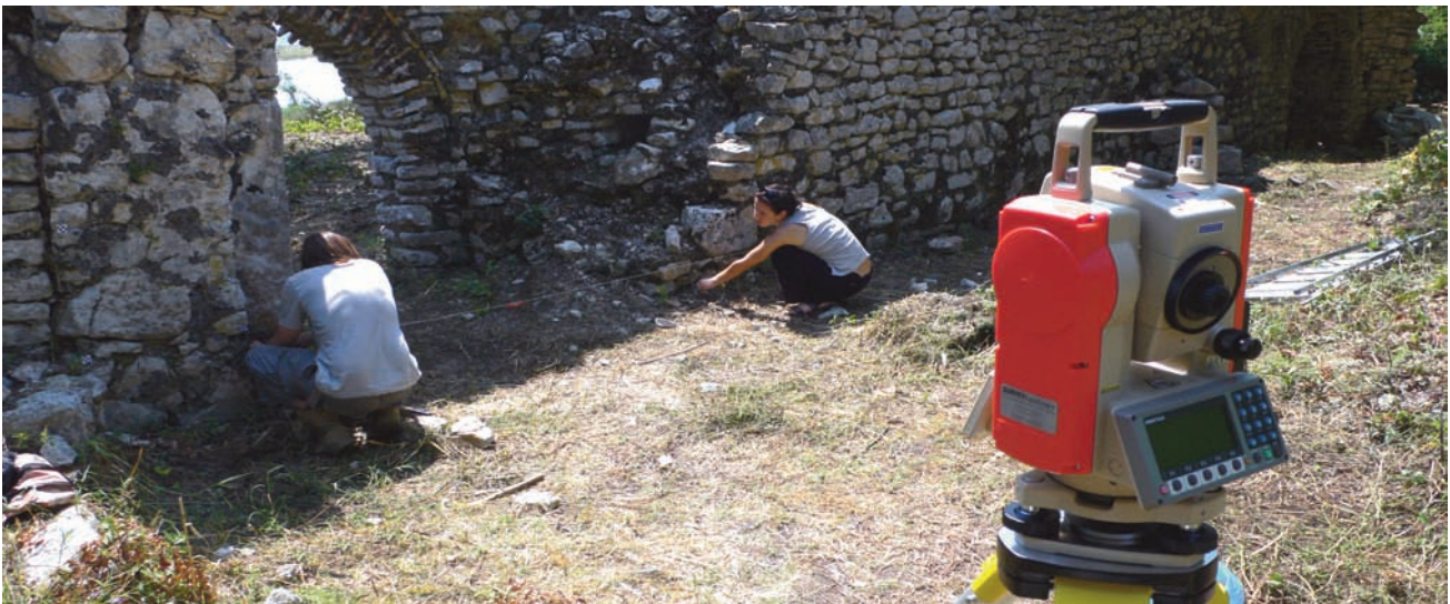
Establishing a survey grid of 3-D reference points for photogrammetric recording of the Water Gate.
