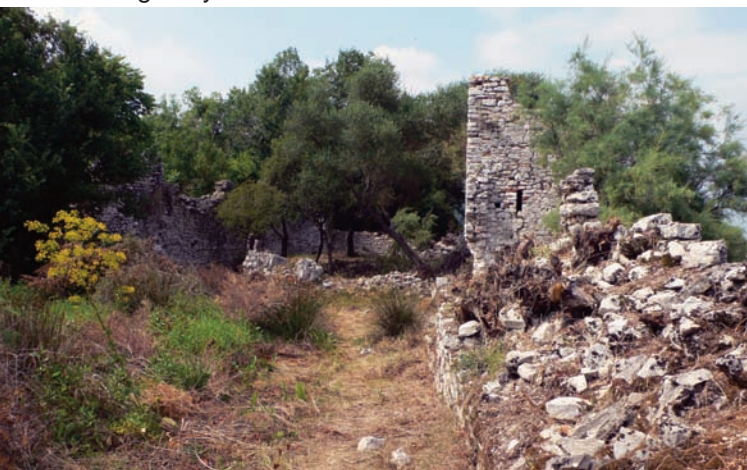
Vegetation clearance from walls and paths on the lower city fortifications.
