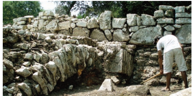
The Bridge, abutting late antique masonry and 10th-century wall.
