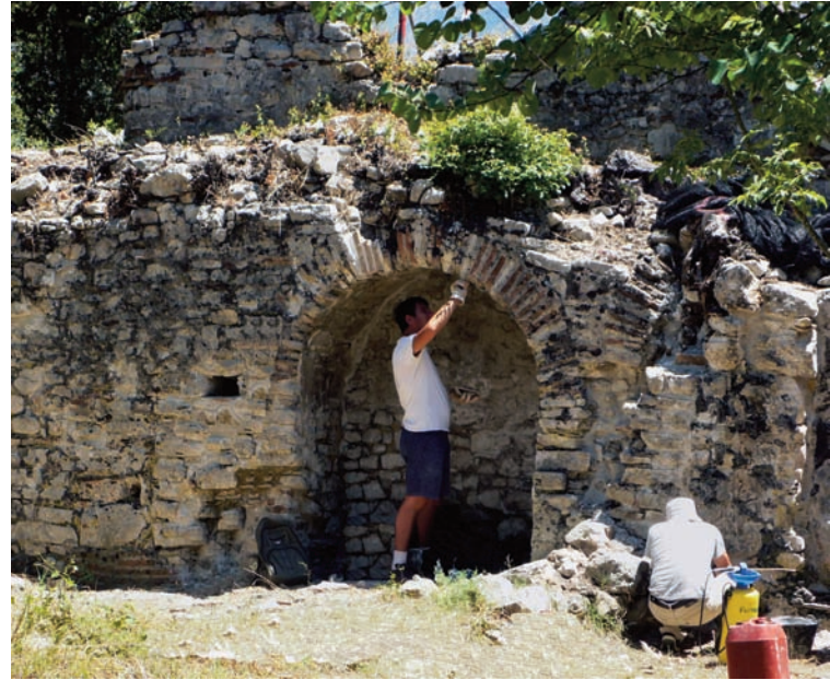
Masonry conservation training initiative at the Water Gate.
