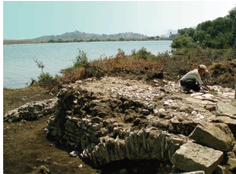
The first span of the Roman Bridge showing the paved surface.
