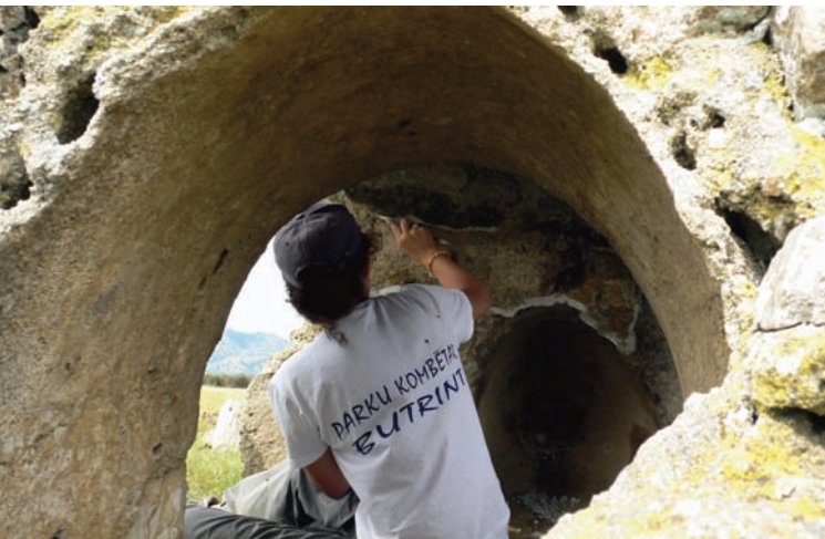
Consolidating plaster on the interior of the Vrina Plain Cremation Tomb.
