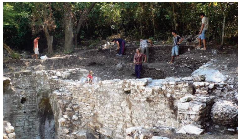
Backfilling and landscaping the excavations behind the consolidated walls at the Well of Junia Rufina.
