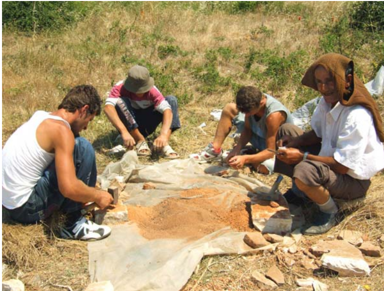
Local workers making ceramic powder for conservation mortar mixes.
