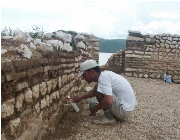
Fig. 27. Conservation of wall plaster at Diaporit.
